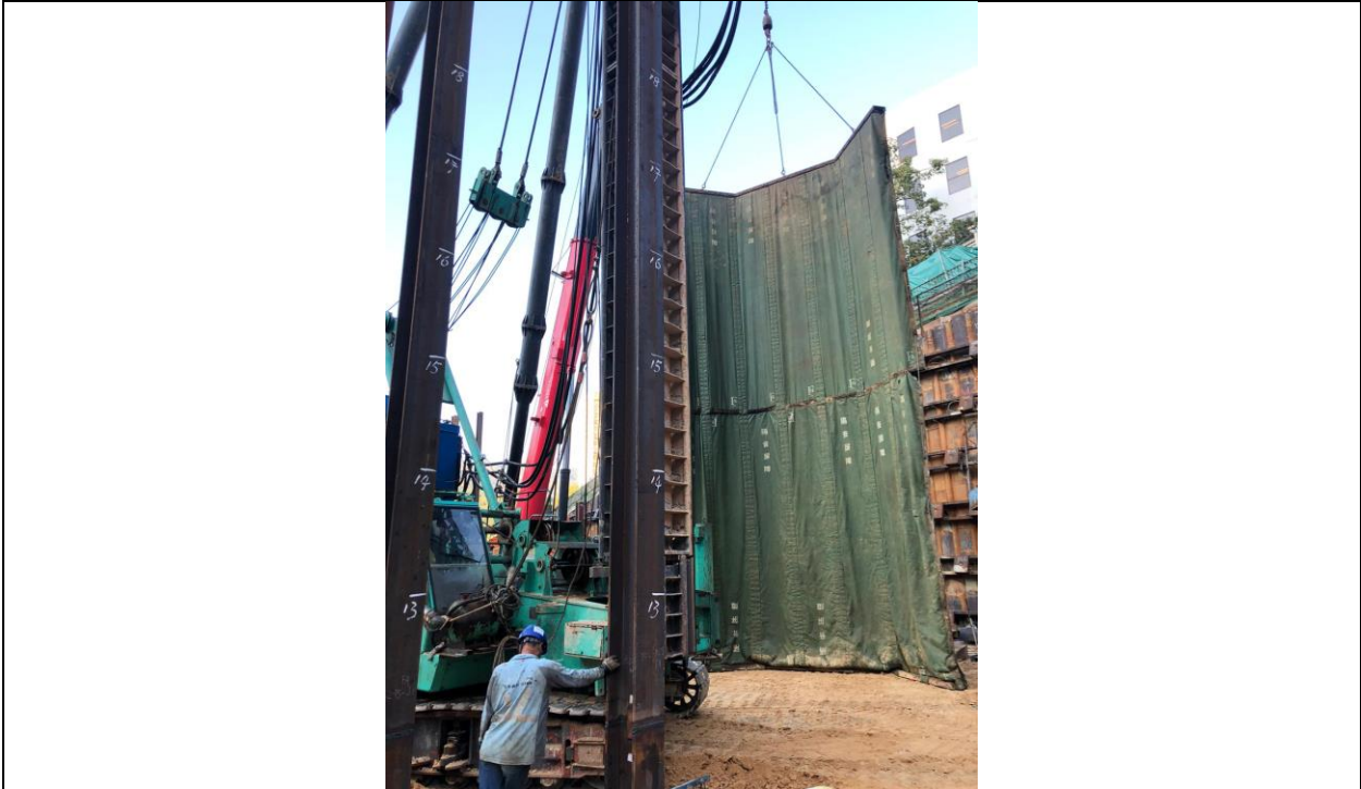
Hoisting of noise barrier during piling
